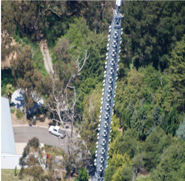
RFS 662 dual polarisation VHF Band III antenna panel
